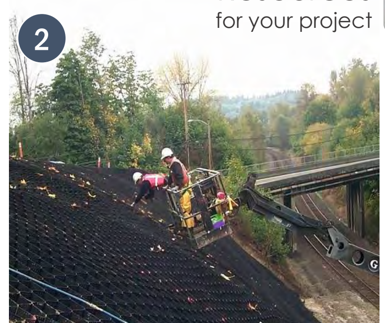
Embankment Stabilization
