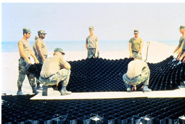
Geoweb being laid at JLOTS II in 1983
