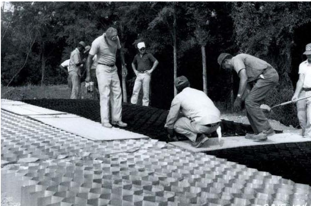
Side by side cost/performance testing of a plastic geocell (termed "roadbase") and aluminium geocells at The Waterways Experimentation Station, Vicksburg, Miss. Circa 1979.
