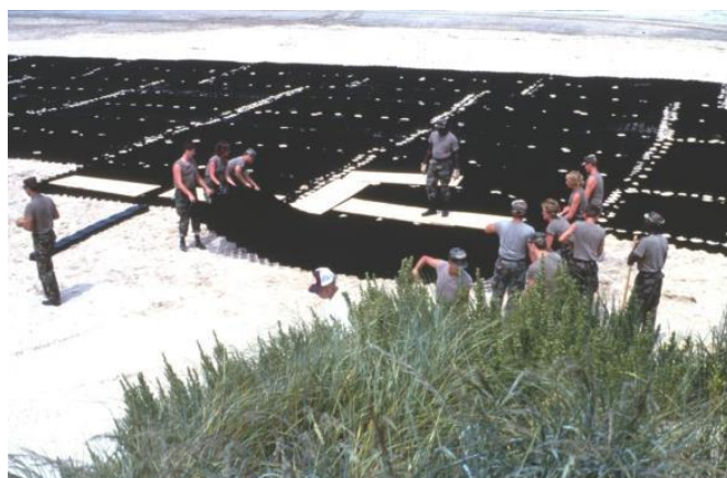
Geoweb being laid at JLOTS II in 1983
